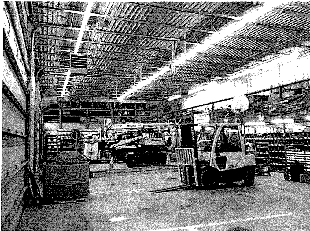
Figure 4b: Milford AWC - existing lighting in garage lighting replaced with new high performance reduced wattage lamps and ballast fixtures with reflectors.
